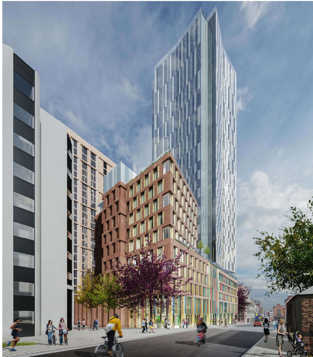
THE MERRION PROJECT - LEEDS | 06.08.20
